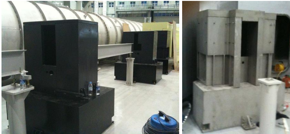
2010.02 Chopper Shielding Install.
